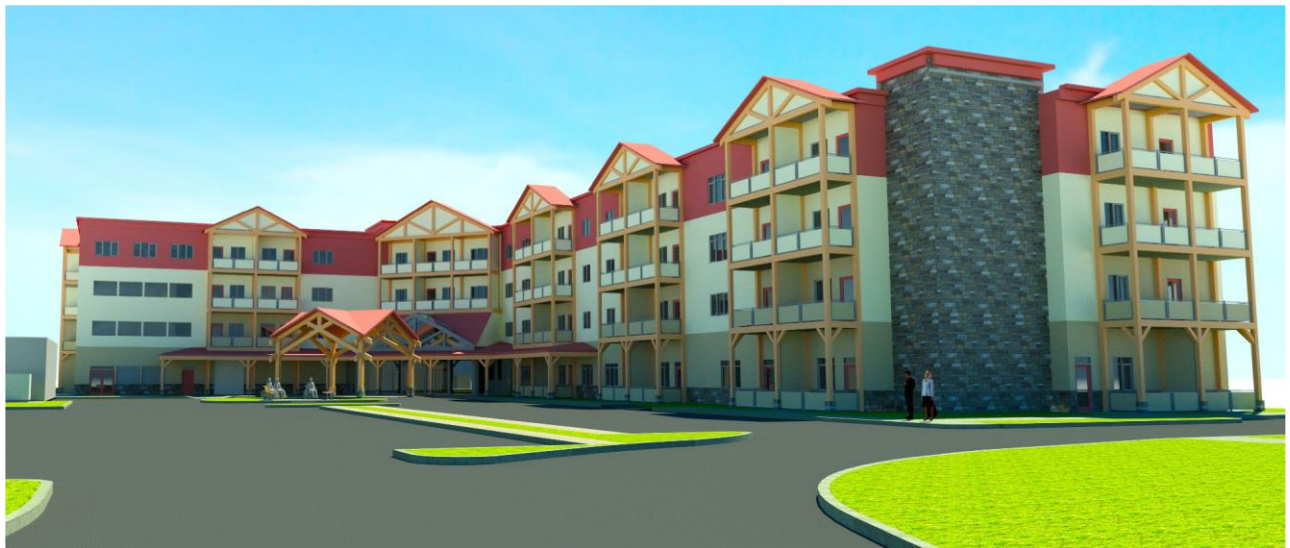
Image of the building (view from Braidwood Road)
